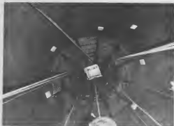
Inside process stack, looking up. Schoorsteen di Process, mirando arriba.
